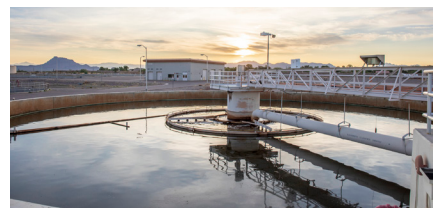
Val Vista Water Treatment Plant Mesa, Arizona (1975)
