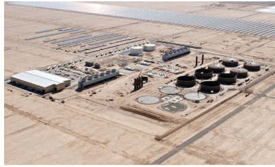
SOLANA SOLAR 280MW Solar Facility in Gila Bend, AZ.
