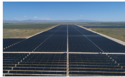
PLEASANT VALLEY 261MW Solar Facility in Ada County, ID.
