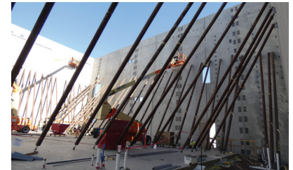
Confidential PHX05 CO-LOCATION DATA CENTER
