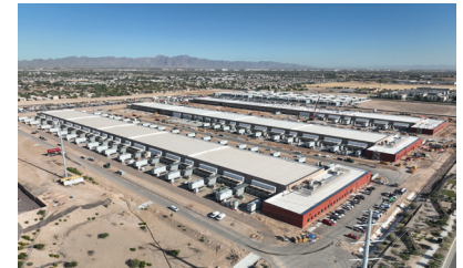
Confidential HYPERSCALE DATA CENTER & MISSION-CRITICAL CAMPUS
