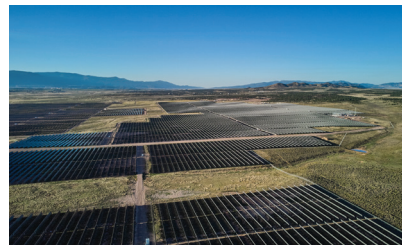
APPALOOSA 240MW Solar Plant in Cedar City, UT.
