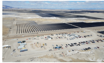
DESRI HORNSHADOW PV PLANT A combination of two co-located photovoltaic facilities with a combined capacity of 360MW and a common substation in Emery County, UT.
