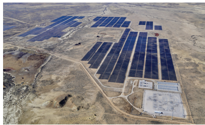
DESRI ARROYO ENERGY CENTER 950MW Solar Plant in Pueblo Pintado, NM.
