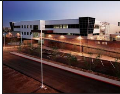
The Operations and Maintenance Center is the nerve center of the entire light rail system.
