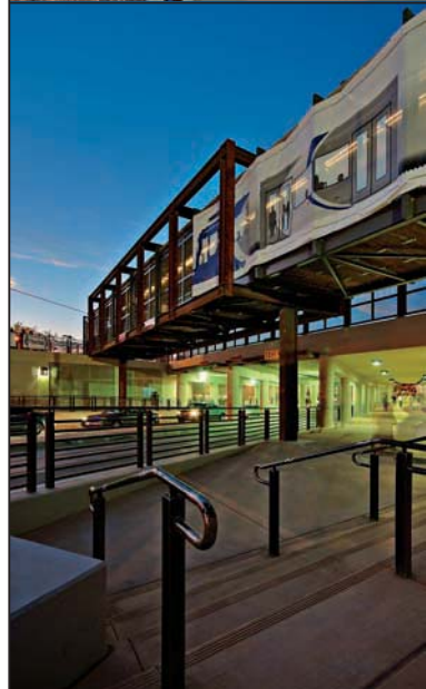
Two widened vehicle lanes plus new pedestrian walkways and bicycle lanes pass under the new pedestrian bridge.
