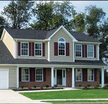
Top and above: Completed military family housing from Phase One at McGuire Air Force Base
